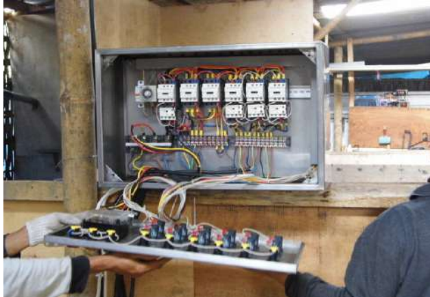
Gambar 14. Panel Listrik Proses Pencucian Garam Basah
